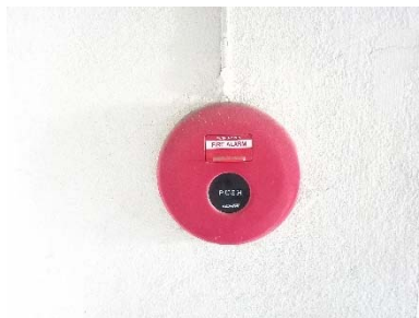
Fire Alarm Manual Station
